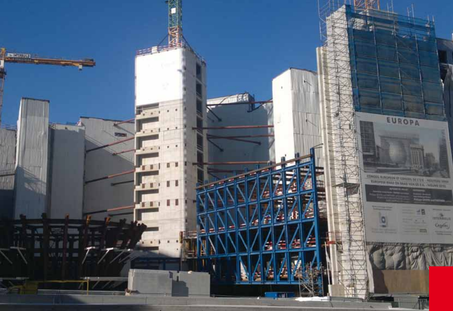
The new “EUROPA” building for the European Council still under construction
